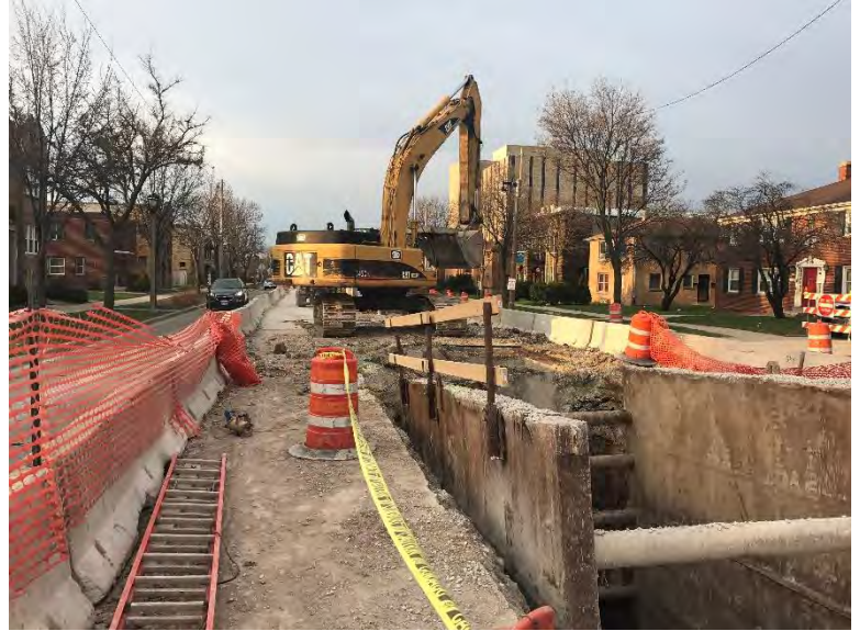
Constructing box culvert on 27 th Street
