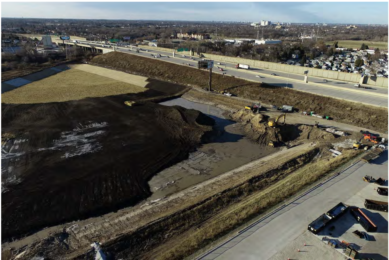
Construction of the flood storage basin.
