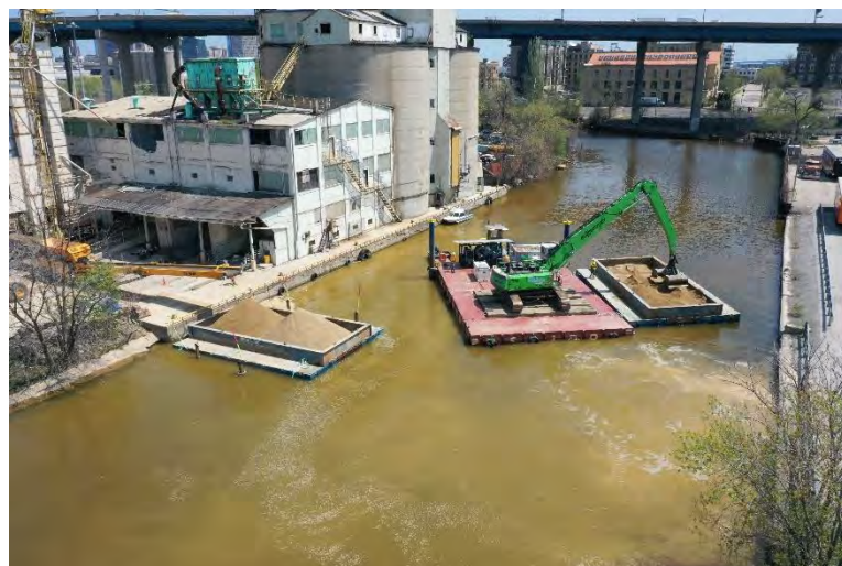
Placing fill for the wetland base at Burnham Canal.
