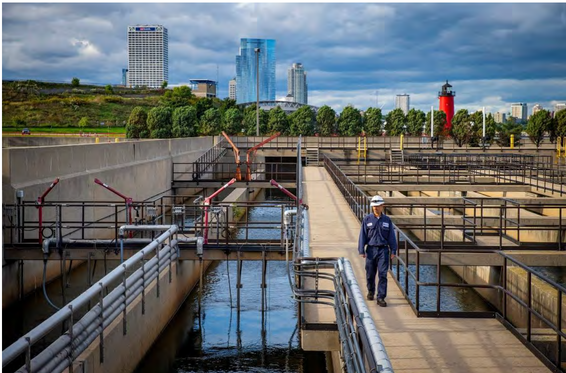
The majority of the operating budget is targeted towards operations of the wastewater reclamation facilities, as seen above.
