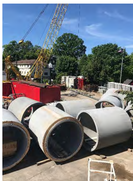
72-inch diameter sewer to install as part of the project.
