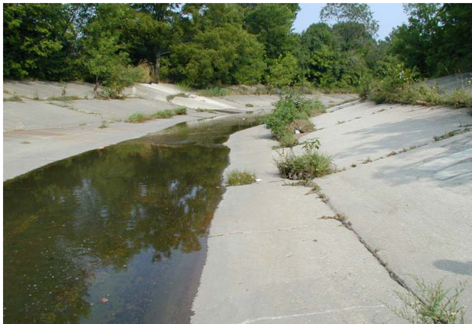
Figure 4. Honey Creek - Concrete Lined Channel; low-flow invert and sidewalls.
