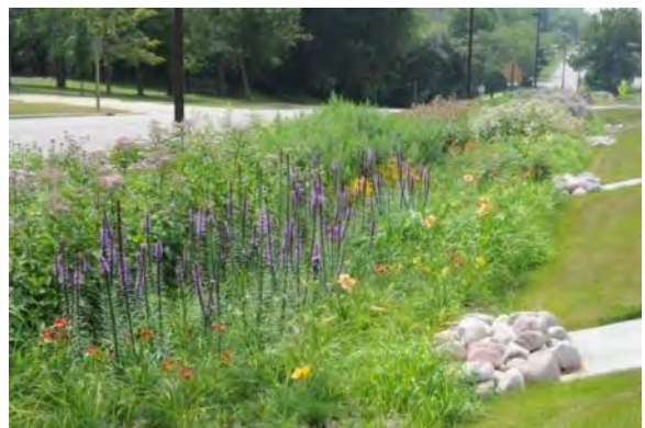
Figure 2-14. Bioswales (Greenfield, Wisconsin)
