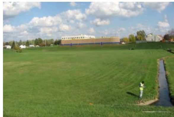
Figure 2-22. Detention Basin (Matteson, Illinois)
