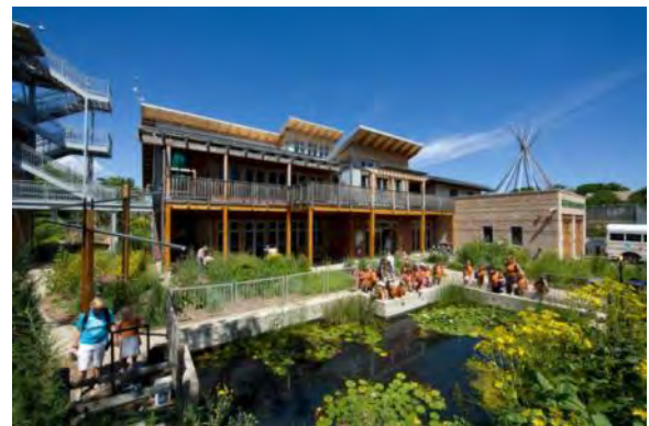
Figure 3-14. Example of Environmental Learning Site (Urban Ecology Center, Milwaukee)
