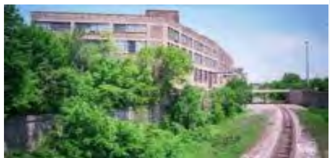
Figure 1-3. Esser Paint Building and Railroad Tracks
