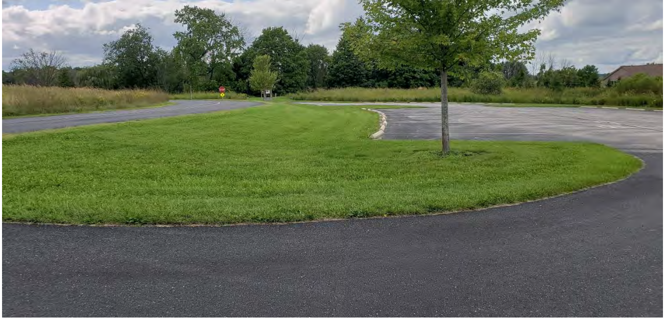
Potential Parking Lot BMP - 40A, Leonard J Yahr County Park
