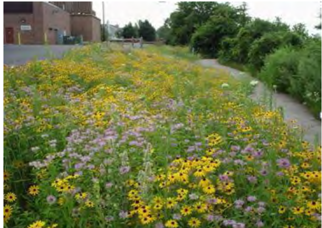
Filter strip along municipal building in Algonquin, IL
