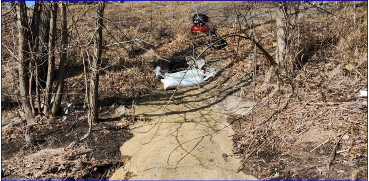
A view of the outfall after the impacted was cleaned on 03/12/25
