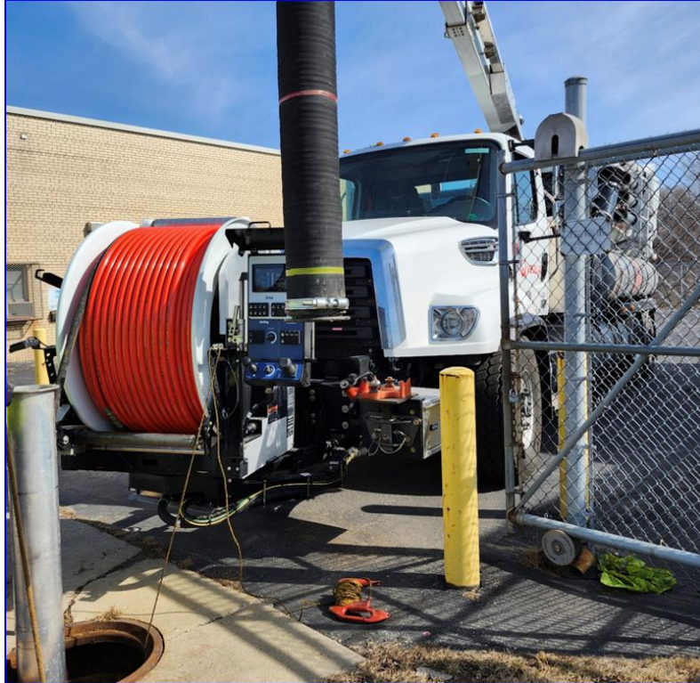
Veolia crew cleaning the impacted sewer on 03/12/25
