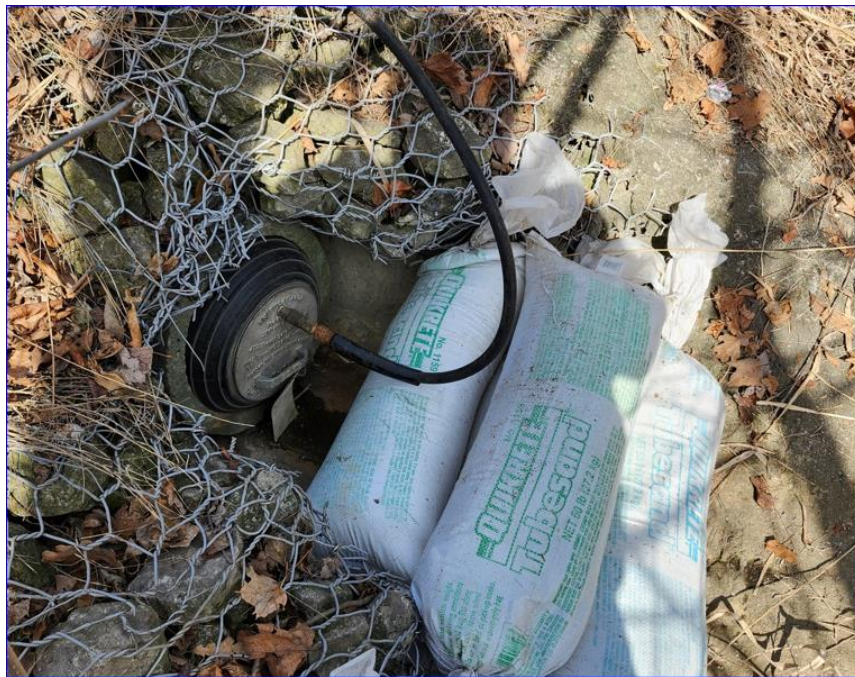
Sewer Plug and Sandbags were used during line cleaning on 03/12/25
