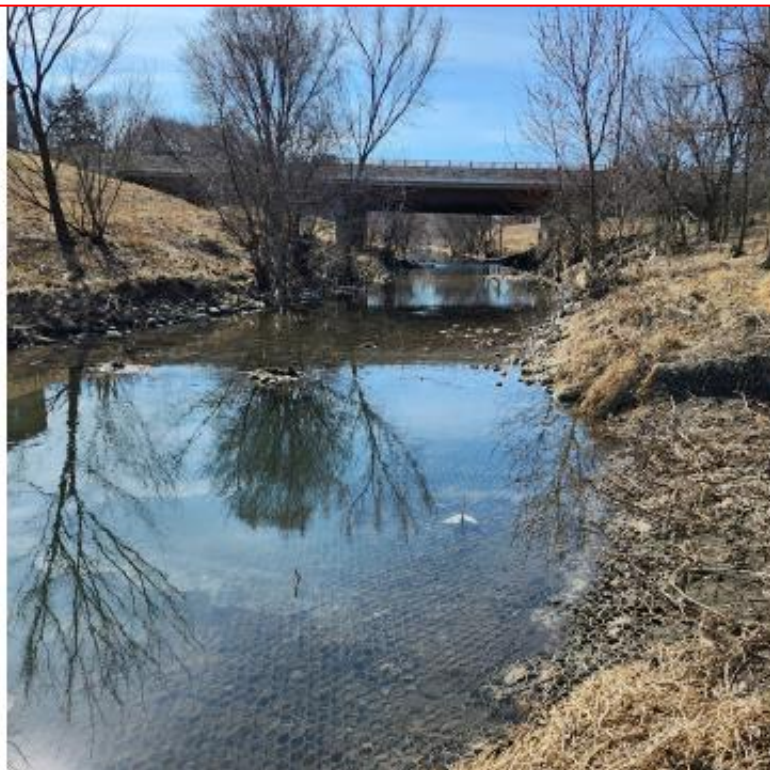
Photos of Lincoln Creek after the incident
