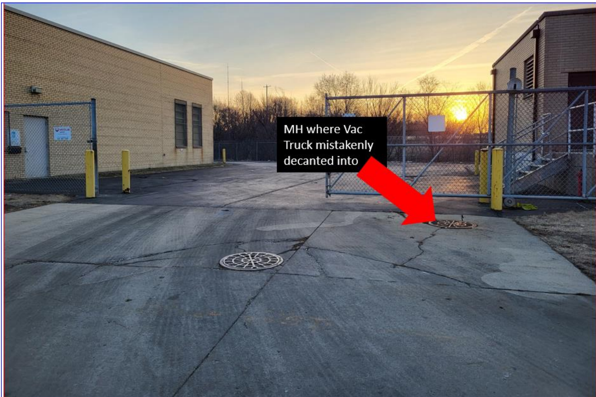
Manhole where Vac Truck decanted into
