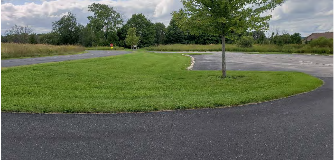
Potential Parking Lot BMP - 40A, Leonard J Yabr County Park
