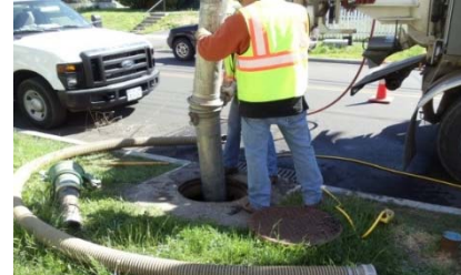
Some GI maintenance builds off or replaces maintenance already being performed in our region - for example inlet cleaning and parking lot cleaning.
